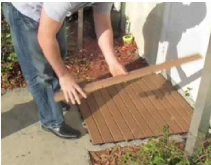
The Edge-Perfect edging will not run past the corners of the tiles, they will be set flush with the tile's edge. When edging is completely installed we supply corner tiles that will snap into place also using the same male/female technology as the deck tiles and the Edge-Perfect edging.
