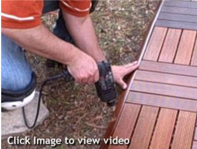
**For installation on cement:** Secure to the foundation using concrete screws (Tapcon blue screws in most hardware stores). Any size screw you prefer can be used, but our recommendation is Philips head 3/16" x 2-3/4" for a good hold that will withstand repeated foot traffic.
