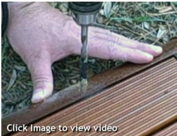
Using a drill bit size recommended by the screw manufacturer (e.g., with the Tapcon 3/16", they recommend a 5/32" bit), pre-drill the edging downward all the way through in two places with the same size wood bit. Make sure the holes are evenly spaced from each other and the ends of the edging for aesthetics.
