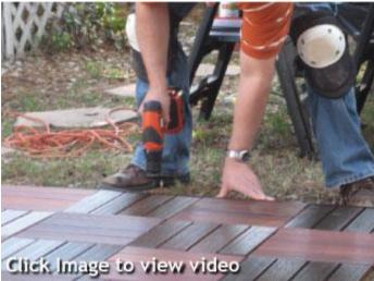
For aesthetic appeal, either purchase wood plugs from a local hardware store for the counter sunk heads, or paint the top of the screw with a brown outdoor paint.
